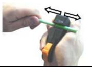
Keeping the it closed, pull the stripping tool with jacket and remnants of the shield off the end of the cable.
