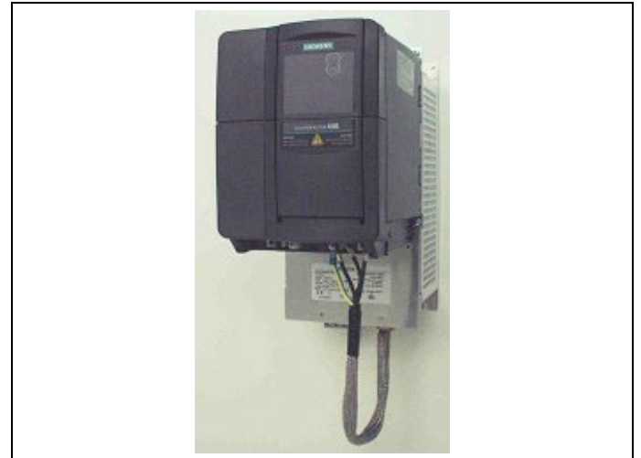
Fig. 5 Sub-chassis: LC filter, Size B
